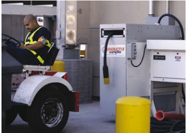
The PLB400 can be used with with any model of 400 Hz converter; shown here mounted next to the converter.
