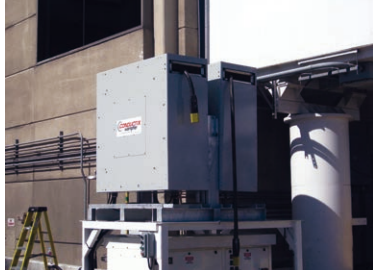
PLB400 mounted at the tarmac level and suspended above the converter.
